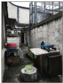
图13 乱搭乱建现状 Fig.13 Chaos and unauthorized construction
